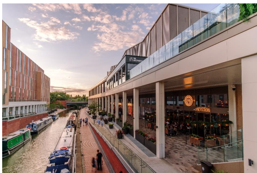
Images above: completed Castle Quay Waterfront development
